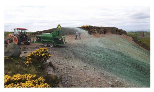
We have three hydroseeding machines which allow us to cater for small, medium, and large sites. These are all suitable for areas that are inaccessible to standard horticultural machinery.
